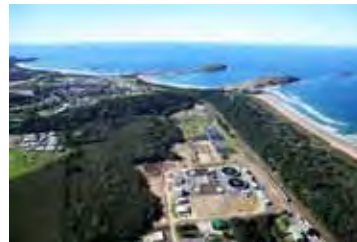
Water Reclamation Plant
